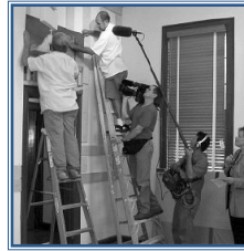
TFA's film crew captures Daniel Lechón and Cesar Rivas installing a panel at the Kenedy Ranch Museum
